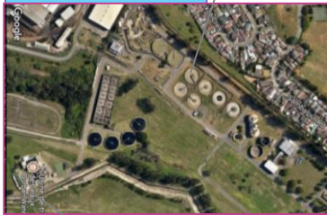
Durban Water Recycling Plant
